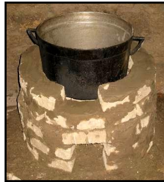
Figure 17: Window and Mortar on the 5th layer
