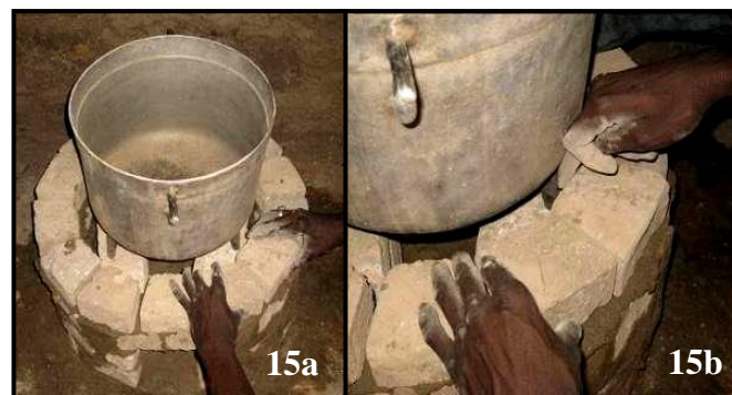
Figure 15: Adjusting the 4 th layer to the pot
