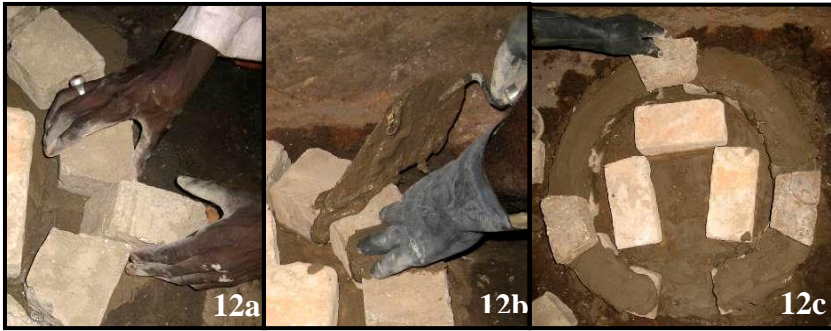
Figure 12 : Finishing the first layer
