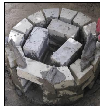
Figure 14: Completing the 3 rd layer of bricks
