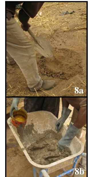
Figure 8 : Mortar preparation
